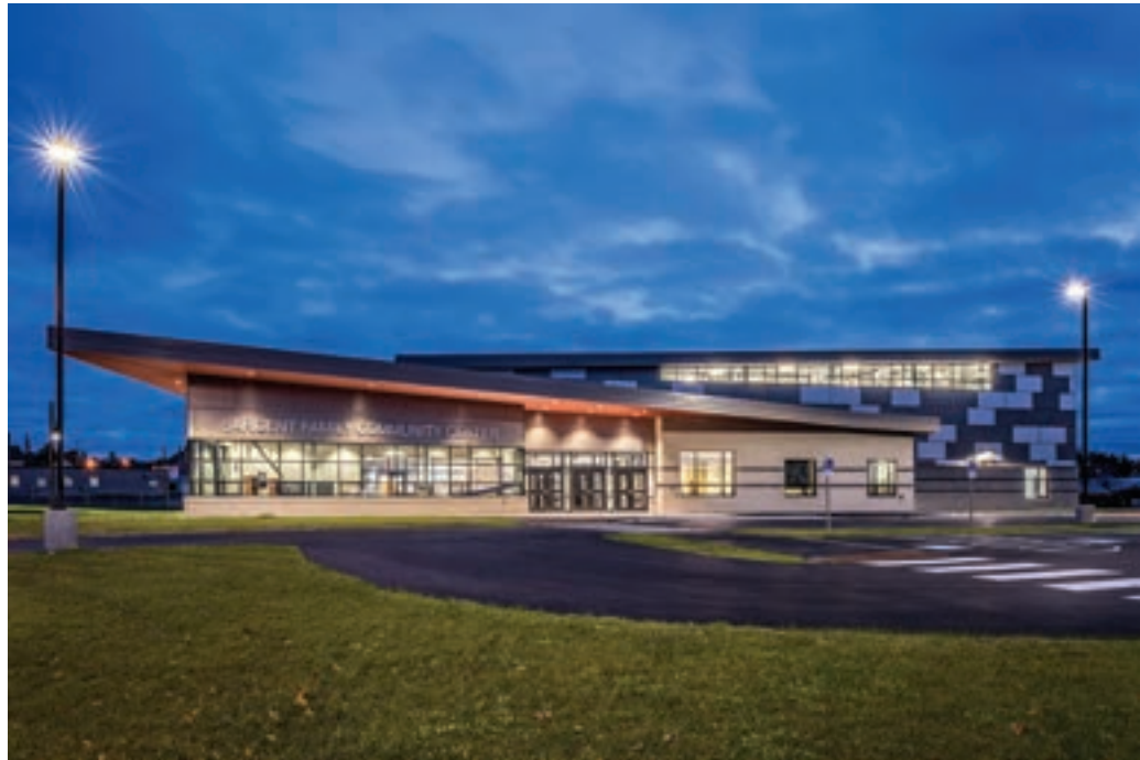
The Presque Isle Community Center, designed by architect Judy Johnson, is a beacon for community engagement within the city. It includes a 30,000-square-foot recreation center with a gymnasium and indoor walking track, teen center, senior center and art center.
